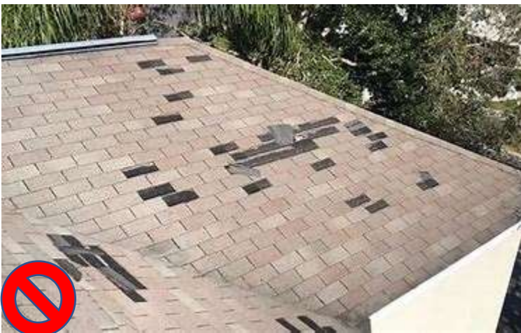
Roof with missing shingles
