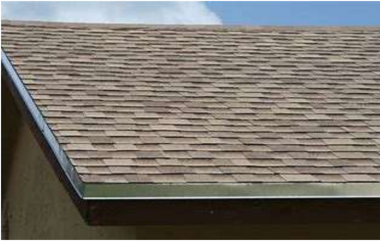
Roof with no missing or mismatched shingles
