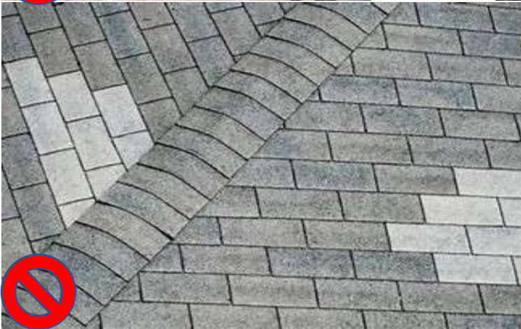
Roof with mismatched shingles
